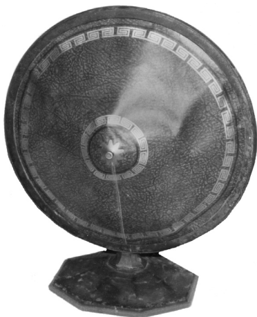
CROSLY MUSICONE – Manufactured by the Crosley Radio Corporation of Cincinnati, Ohio, in 1925, this paper cone speaker is the "Regular Musicone." It is 12" in diameter and sold for $12.50. There were also other Musicone models — the "Super" and the "Ultra" models. (Clark Trissell – Lincoln, NB)
